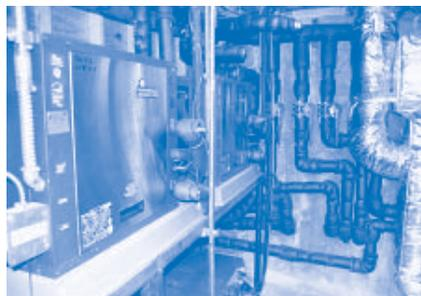
*Three of the seven ground-source heat pumps. Black insulated lines go to the ground loops in the 14 borings*
