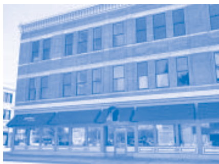
Above the commercial space on the ground floor, Lantow Lofts brings seven market-rate condos with numerous amenities to downtown Rockford.
