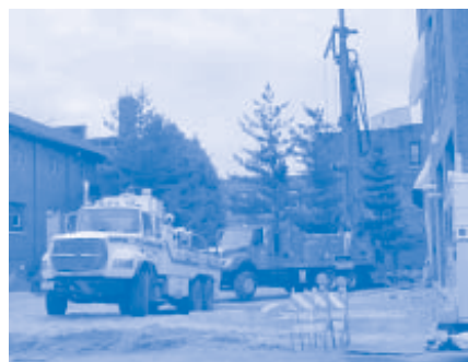
Drilling for the geo-thermal ground loops - 14 borings each at 300 feet deep.
