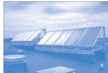
*Solar panels on roof send heated fluid to heat water in basement tanks.*
