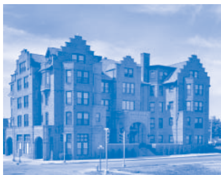
New Holland Apartments, Danville, Illinois
