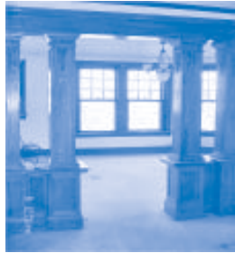
Beautiful woodwork was preserved in residential units.
