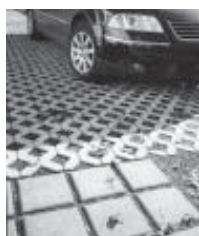
“Grasscrete” allows runoff to be absorbed into soil.
